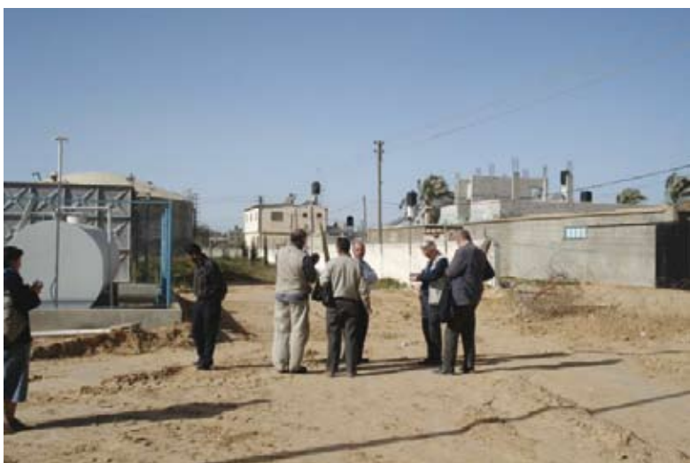
18b European Hospital, Khan Yunis. Area where bomb fell and Damaged hospital generator. 31.10.2009. Photo by SVA
